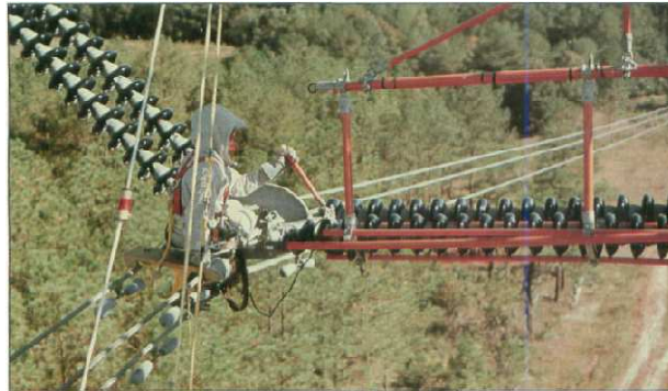
Figure 2: A Linemen Wearing a Conductive Suit is About to Change a Insulator String
